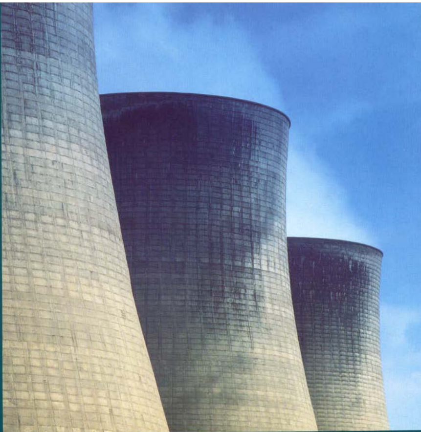
Above Steam rising from giant cooling towers.
